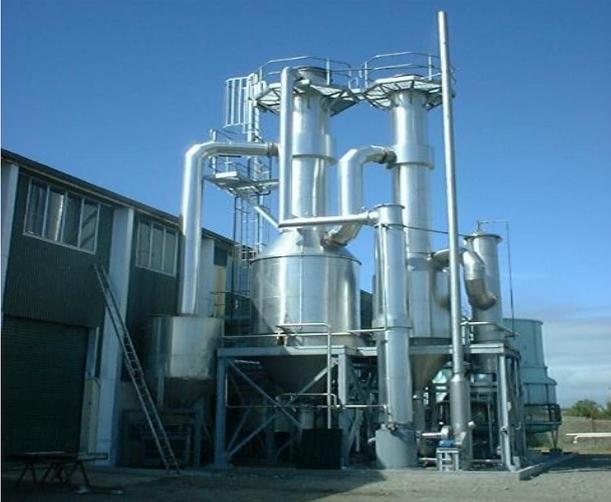
**Rendertech** evaporators, when used in rendering and fishmeal industries, maximise the return from raw materials, increase plant yields and eliminate a high strength wastewater stream. The plants are simple to operate and maintain.
